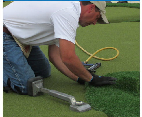
Install the pre-cut turf and fringe.
