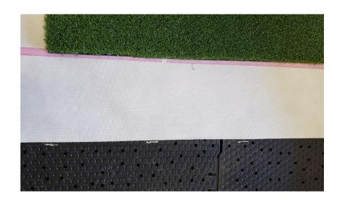
7. When creating arcs or curves it will be necessary to overlap your seam tape to create the desired shape.
