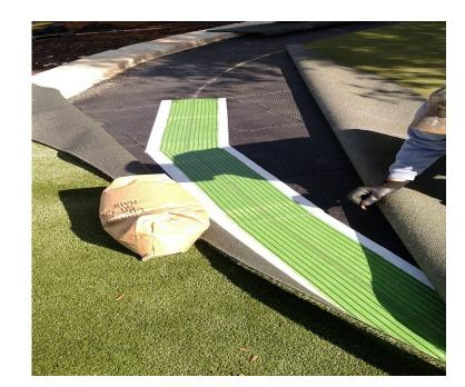
8. If using tubes of Turf Claw MP trim tip of tubes. Do not hold tubes of any adhesive directly over the turf. Having a cloth, pail or cover to work over is important. Glue on synthetic turf needs to be wiped off immediately with a clean cloth. Any glue on turf will be a problem but excessive glue must be removed immediately with a cloth and alcohol or a product like Goof Off. Protecting your turf is essential.
