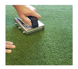
13. If you need to adjust your seam for a final fit now is the time. Turf Claw MP will grab in a few hours and takes 24 hours for a complete cure so you will have time to reposition.
