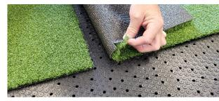
3. Trim/cut turf to fit. For straight cuts you can row cut or you can mark with a chalk line and cut with a straight edge.
