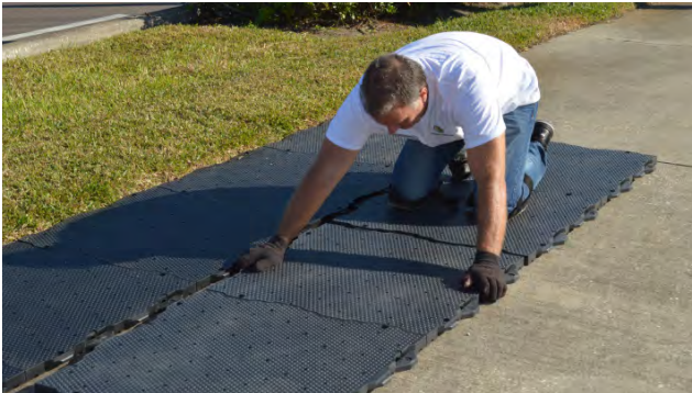
Sliding 2 Panel Sections Together
