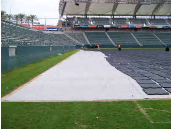
Geo Fabric Ready for More Panels
