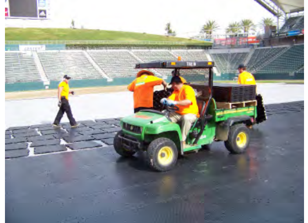
Moving New Pallets of Panels on Installed UBS Panels
