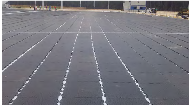
Pre-assembled Rows of 12 Panel Sections
