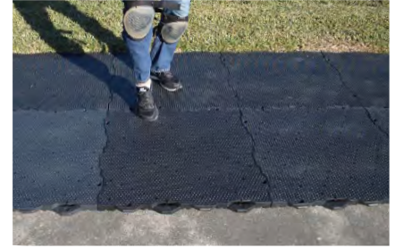
Be sure to adjust installed panel gaps as needed
