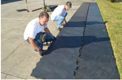
Align the 2nd row in preparation to be zippered
