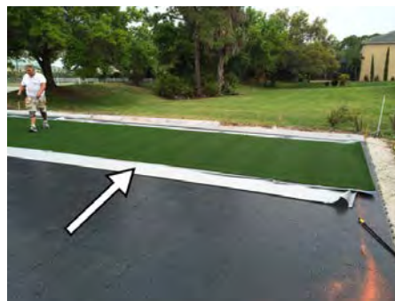
A Geo Slip Sheet is Temporarily Placed Under the Rubber or Felt Backed Turf to Allow for Positioning
