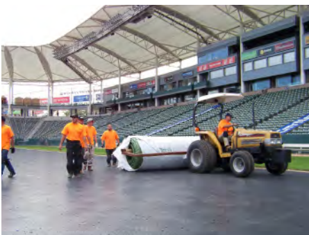
Turf Rolls Moved into Position
