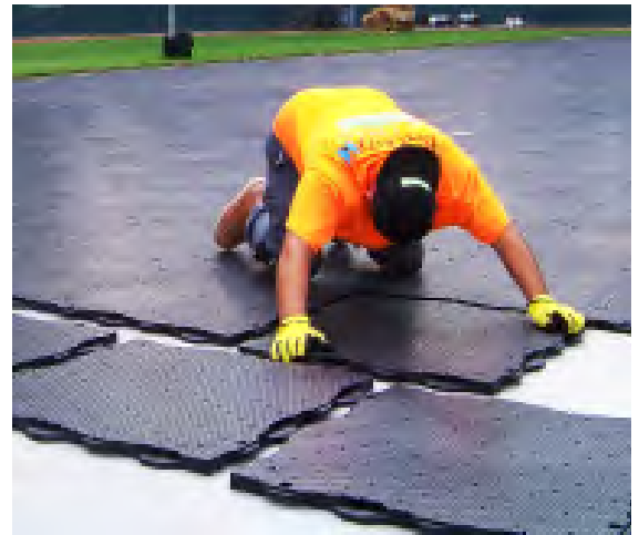
Pulling Panel Technique in Action
