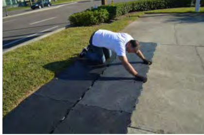
Zipper th 2nd row into the initial string line row
