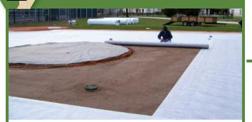
Installing a geosynthetic stabilization fabric helps ensure the stability and regulate drainage in the prepared sub base. Install UBS Panels
